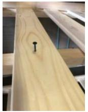
Once you have attached the base slats we need to secure the centre rail to the base slats. Select any central base slat. Then from the top, using fixing E, base slat screw through the base slat into the centre rail. No pilot hole is provided to ensure a tight fitting.
