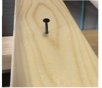
TIP:-When you have attached the base slats you will have additional base slats screws. Out of the 12 slats screw 4 of them directly into the centre rail. Using the base slat screws simply drill through the top of the base slat into the centre rail. This will further strengthen the bed.
