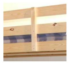
These two rails prevent the guard rails from being forced apart, very important. Using a tape measure find the centre of the back guard rail and centre of the front guard rail. Make a small pencil mark. Then attach each guard rail support to the front using the screws provided. These cover both the two guard rails and secure onto the side rail.
