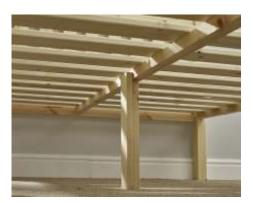
It is IMPORTANT that this is positioned correctly and remains in place while the bed is being used, failure to fix will weaken the bed. This part is manufactured using recycled timber as the component is out of sight. The centre leg will hover slightly off the floor, when the bed is in use it will move down and support the bed. This is to protect the leg if the bed moves.
