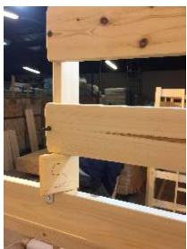
Push the ladder to the headboard in and hook over the top blue headboard facia. Centre the ladder so both the ends of Part E10 and E09 meet the struts. This should be a gap of 79cm from each corner post.
