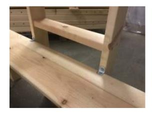
The bottom of the ladder is secured by fixing to small brackets to the top of Part 4E - thick bottom facia.
