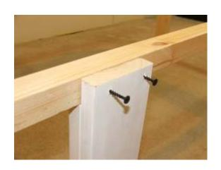
The centre leg is located under the centre rail, in the centre. Simply measure to the centre of the bed and locate under the centre rail. Using two black screws attach from the side. (These are self threading screws so no pilot holes required)
