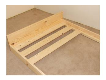
Step 3. Now get the base slats and space evenally along the bed. Make sure the base slats butt in on one side rail, then screw in. Go to the opposite side and locate the centre
